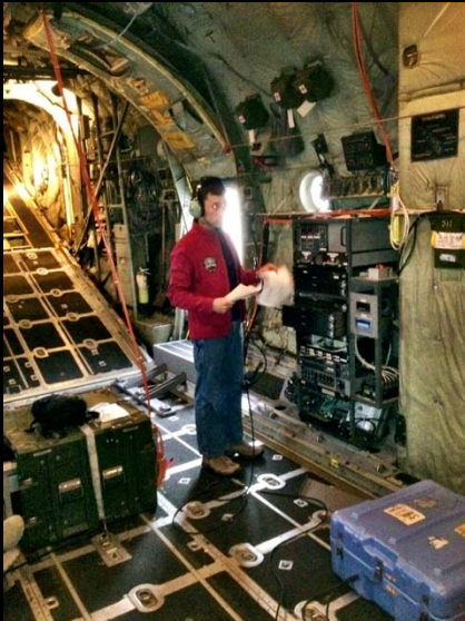
A Data Acquisition Rack
